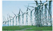
风力发电站 Wind Power station
